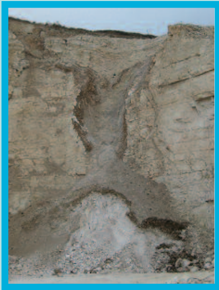
Fig.1. The large pipe in Flixton Quarry - View north.
