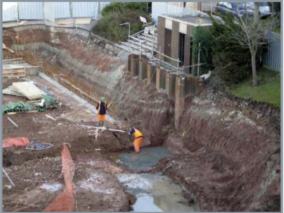
Figure 3. GeoExposures web site example showing the Upper Triassic Branscombe Mudstone Formation exposed in the excavations for the William Smith Building, BGS, Nottingham in 2008.
